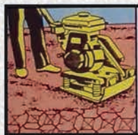
Vibrate the Laid Surface with fine River Sand
