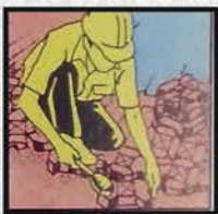
Lay and Interlock Paver Blocks
